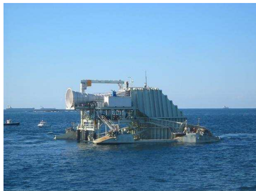
Figura 2.4: Central Energetech - Vista lateral.
