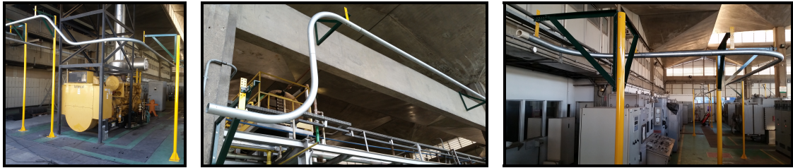
Figure 1.8: Installation of DORIS rail system in a utility plant in CENPES.
