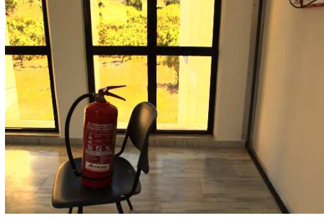
(b) Fire Extinguisher.
