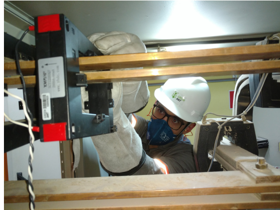
Figure 3.5: Installation of a current transformer by an electrical engineer on an appliance energy supply.
