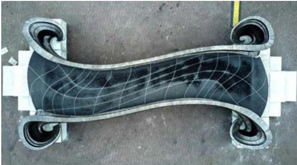
Figure 2.5: World's first metal 3D printed bridge [35].
